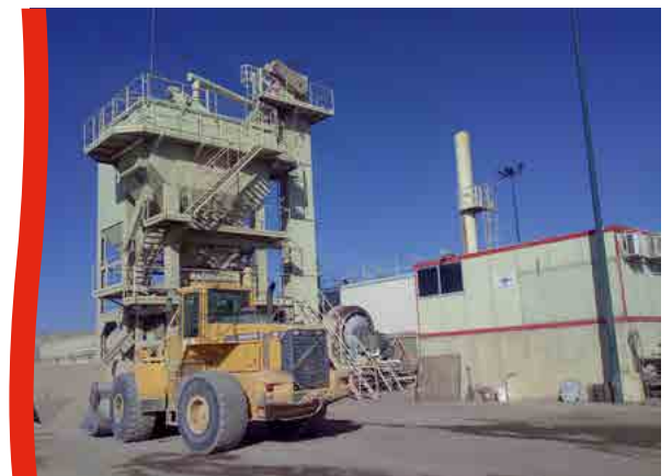
Asphalt mixing plant
